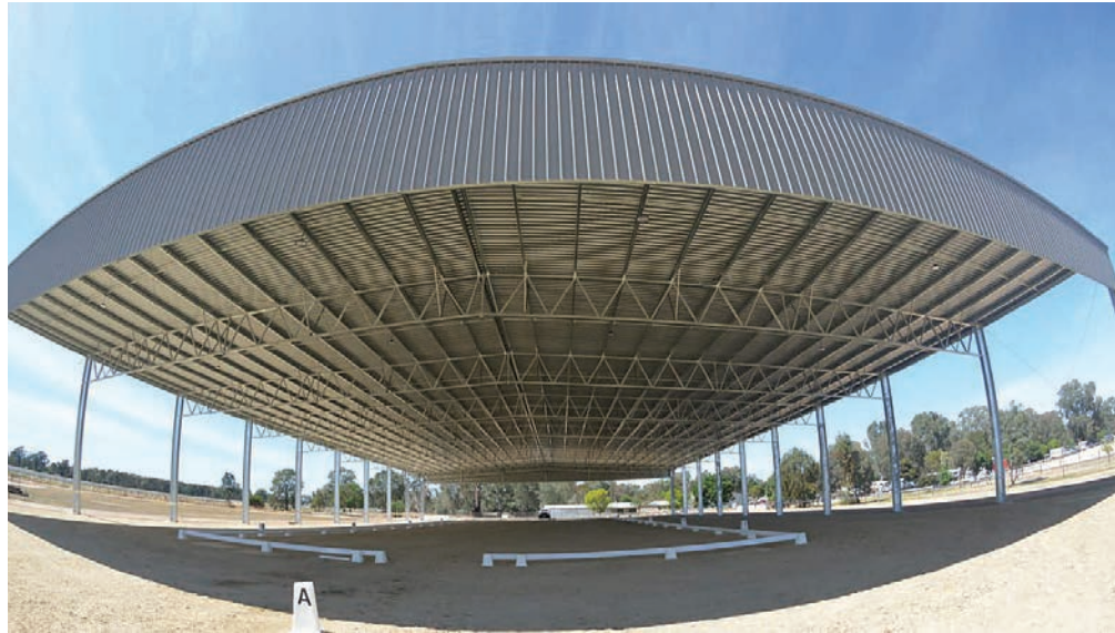
The picturesque Benalla Sports and Equestrian Centre boasts high quality infrastructure including a 72 m x 40 m covered riding arena, providing an all-weather surface with floodlighting for local and regional equestrian participants alike.
