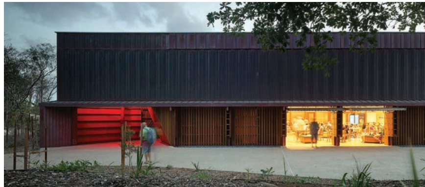
Mon Repos Turtle Centre. Responsible Wood certified ariaply (in Ebony and Natural Hoop) and a glue-laminated timber structure sourced with chain-of-custody from Austral Plywoods and Hyne Timber. Architect: Kirk Studio. Structural Engineer: Arup. Building Fabricator: Hyne Timber. Photographers: Scott Burrows Photographer.
