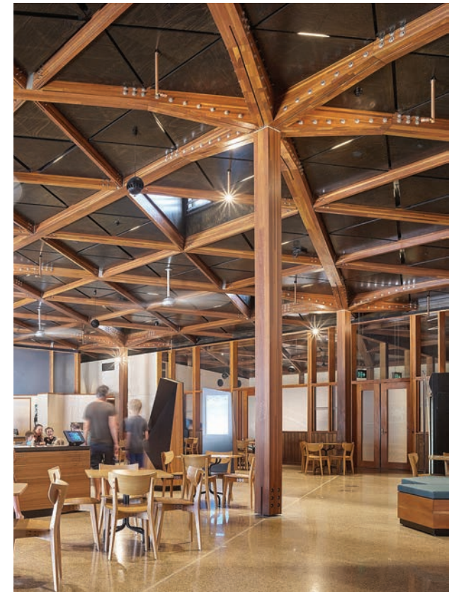
Mon Repos Turtle Centre. Responsible Wood certified ariaply (in Ebony and Natural Hoop) and a glue-laminated timber structure sourced with chain-of-custody from Austral Plywoods and Hyne Timber. Architect: Kirk Studio. Structural Engineer: Arup. Building Fabricator: Hyne Timber. Photographers: Scott Burrows Photographer.
